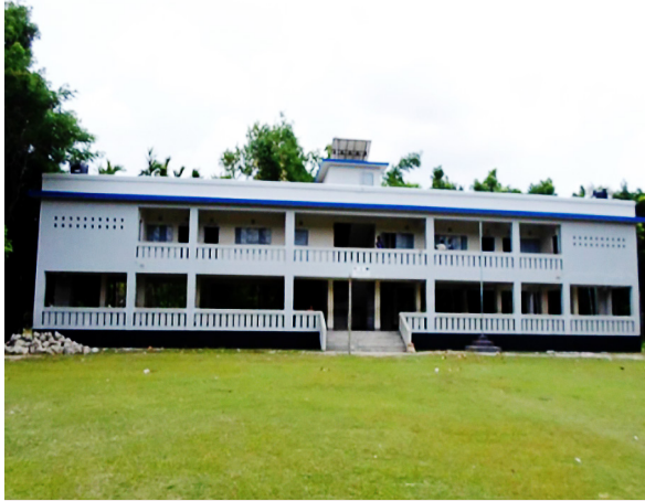
A multi-purpose disaster shelter in Sunamgonj, Bangladesh funded by USAID. Disaster shelters like this one play a vital role in saving lives during extreme weather events linked to climate change.
