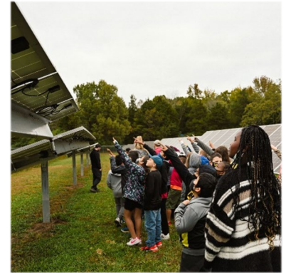
Students in Batesville School District (Batesville, Arkansas) receive a tour of a tracking solar array, which is estimated to be 25% more efficient than fixed panels and excites the next generation about a clean energy future.
